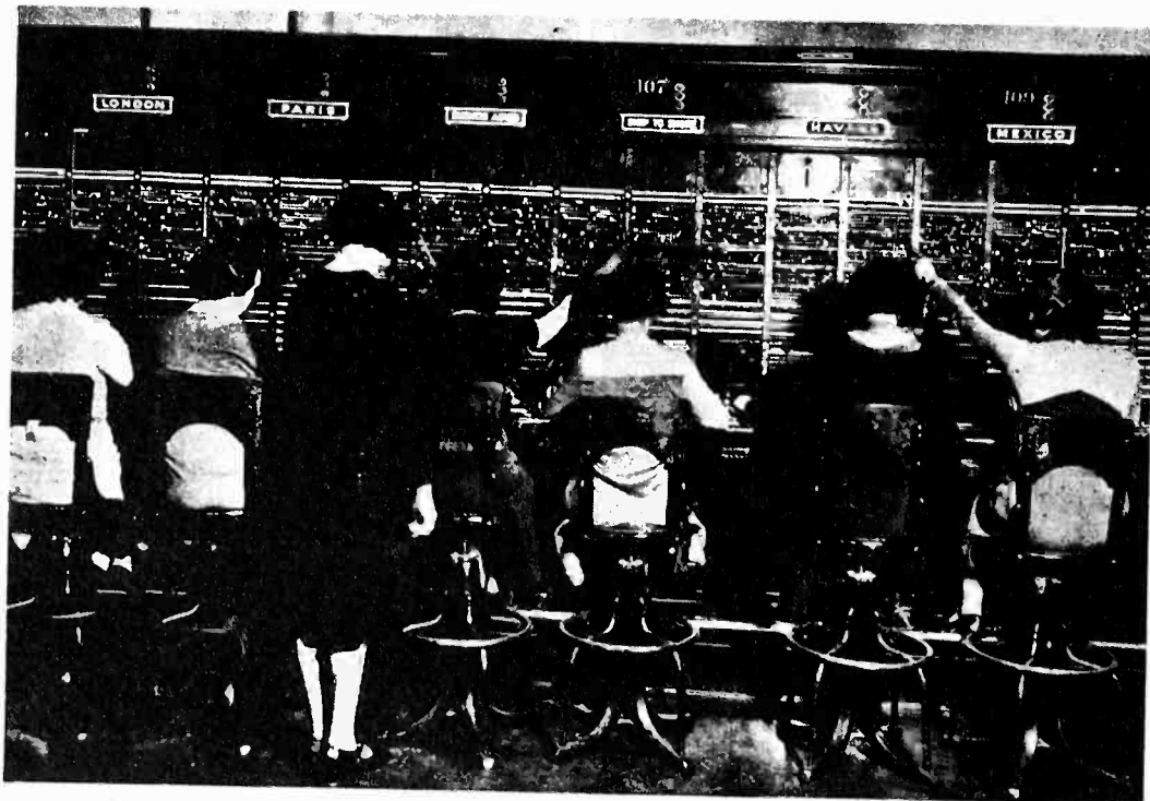
With regular radio telephone service opened last month to South America, now through this short section of switchboard at New York, conversations are handled directly, to London, Paris, Buenos Aires, Havana and Mexico
